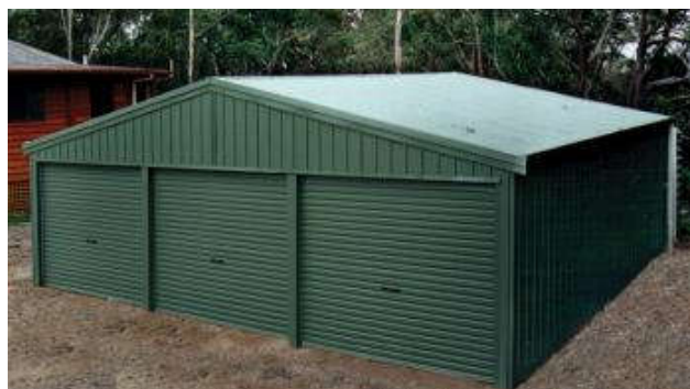
Example of waste management building: Fair Dinkum Sheds NZ
