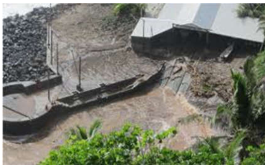
Photo 2. Landslide and debris
