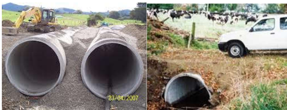
Examples of culverts
