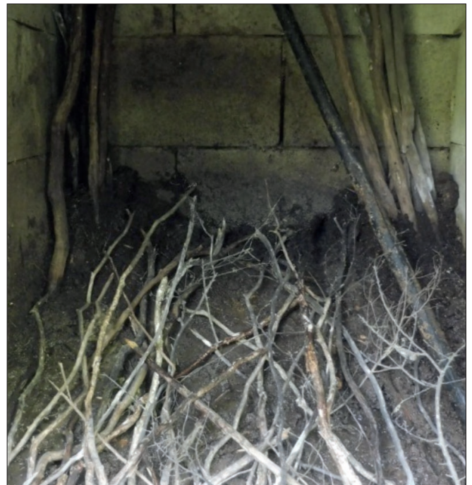
Sticks laid on the floor, and in the corners, of the chamber help air move through the compost. (The black pipe in the photo is from the urine catcher fitted to the toilet pedestal).
