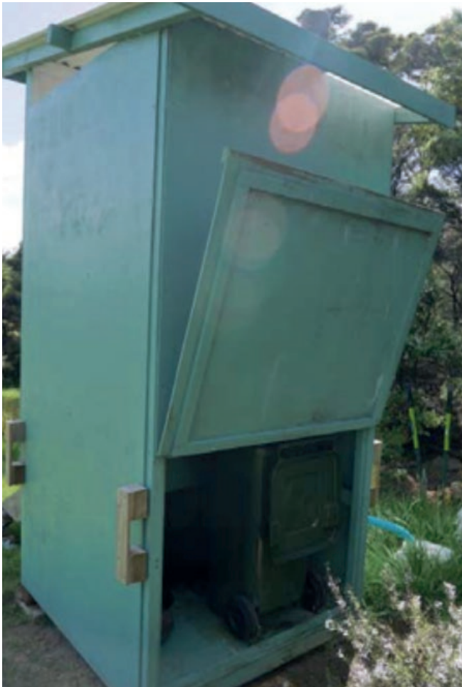
Access to remove the wheelie bin is through a flap at the rear
