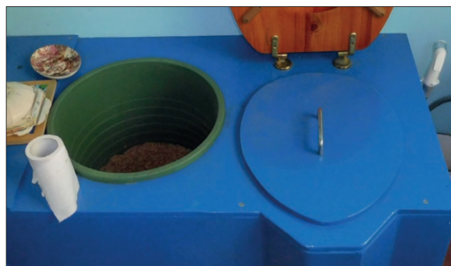
Bucket of Bulking Agent - to add after each use - set into the pedestal framing. This toilet uses sawdust as a Bulking Agent, but any fine, woody material will do.
