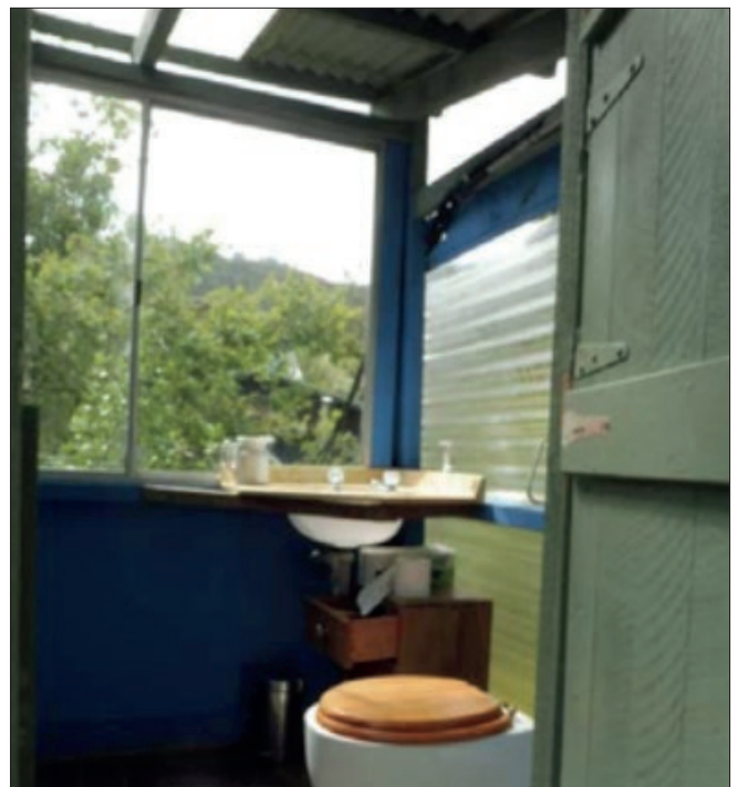
Note the gaps under the roof framing and sliding windows to let the air in; sink for hand washing is in the corner.
