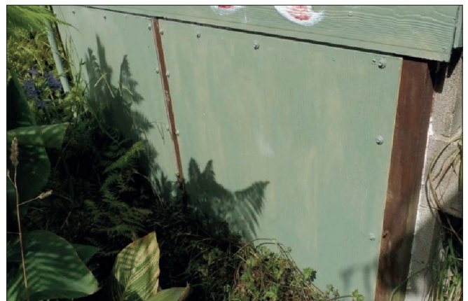
Access hatches fixed with hex-head screws for easy removal and replacement.
