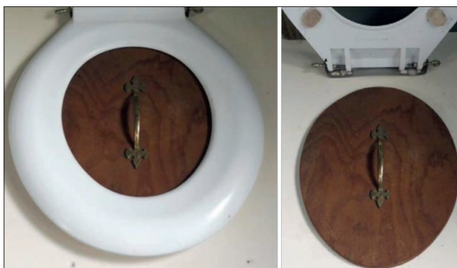
A lid under the toilet seat can keep the chamber sealed well if the seat will not.
