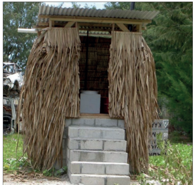
A Kiribati example of using local materials for the toilet room (a local woven mat was used as the door for this example). Note iron roof and gutter for rain water.
