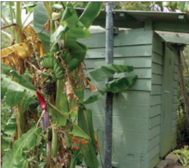
Toilet with bananas planted next to it for the drain, and the black painted vent pipe is shown.
