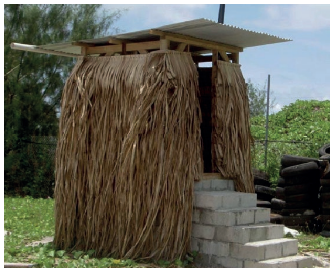
A simple Compost toilet built using concrete blocks, framing timber, roof iron and pandanus leaves.
