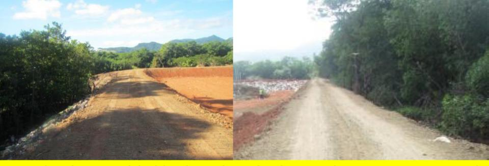
PLACING THE ACCESS ROAD ON TOP OF THE SIDE EMBANKMENTS TO AVOID FLOODING AND WATERLOGGED CONDITIONS
